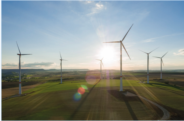
Windpark Wipperfurth (©vsb.energy)
